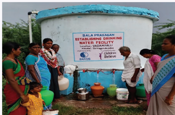
A water tap was installed bringing clean water to Scheduled Tribe Chenchu and Scheduled Caste households.
