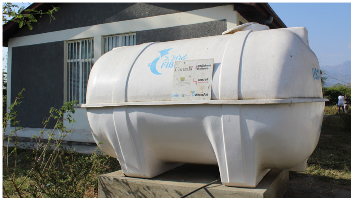
A 10,000-litre water harvesting structure built at a health facility in the project area.
